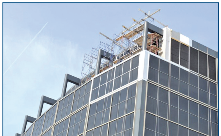
Photo 10 – Pipe scaffolding on setback terraces.
