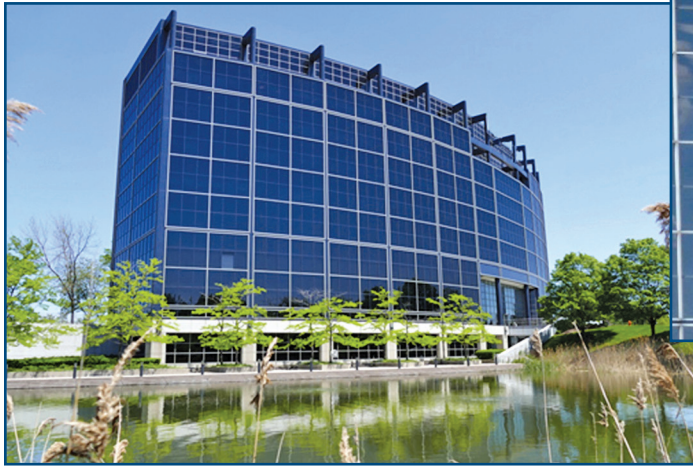
Photo 6 – Overall view of the south and west elevations of the building.
