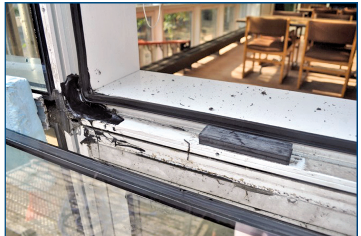
Photo 5 – Repair of internal seals by deglazing.
