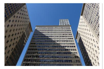
The 3950 North Lake Shore Drive Buildings consist of 3 concrete framed high-rise buildings, all connected at the ground floor by lobby and parking garage areas. The buildings were constructed in the mid-1950s and are all 23 stories tall. The facades of the buildings consist of brick masonry, aluminum framed windows, and metal covers over the window sills. The concrete roof slabs project past the face of the masonry walls at several locations on all three buildings.
