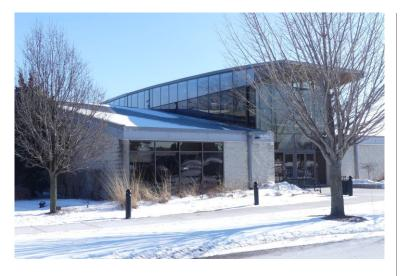
Glenside Public library is a 2-story structure originally constructed in 1982. The library underwent major renovations in 2002, which included a 12,000 square-foot addition. Exterior walls consist of a combination of single-wythe concrete masonry unit (CMU) walls, cavity wall assemblies clad with brick veneer, and curtain wall systems.
