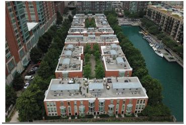
The East Water Place Townhome complex consists of eight 3story wood framed buildings, constructed between 1996 and 1998. Four of the buildings include 6 townhome units and the other four buildings include 8 townhome units, for a total of 56 units. The exteriors of the buildings are primarily clad in brick and stone masonry. The roofs are low-sloped with insulation placed within the ceiling cavity below the roof sheathing. The roofs also include extensive rooftop decks.
