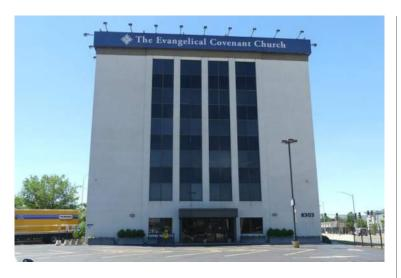
The Evangelical Covenant Church building in Chicago, Illinois is 6 stories tall, and square in plan. The facade typically consists of curtainwall with exposed concrete columns. There are mechanical equipment and a penthouse on the roof. The roof is low slope with a brick parapet around the perimeter. Light fixtures extend from the roof over edges of the building on all 4 sides. The light fixtures are supported by steel framing supports.
