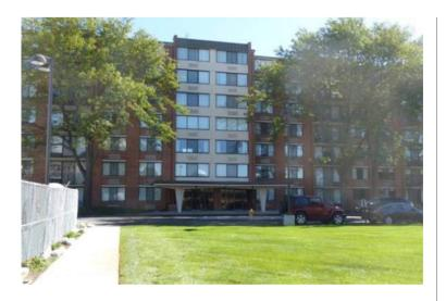
St. Regis Condominiums is a 90-unit residential community located in Lombard, Illinois, which was constructed in 1974. The building is a 7-story structure with cast-in-place concrete floor slabs and columns. A basement-level parking garage extends beyond the perimeter of the building. The roof of the building is low slope with single-ply membrane roofing. BTC had performed several evaluations and restoration projects for the Association in the past.
